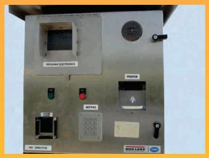
The image shows the kiosk wherein barcode scanner, ticket printer and the weigh indicator are located. It has a voice assisted guidance system for truck drivers and a button system available to cancel / accept the weights, based Remote LED display. The display system inside the kiosk helps the instrumentation person carry out calibration.
